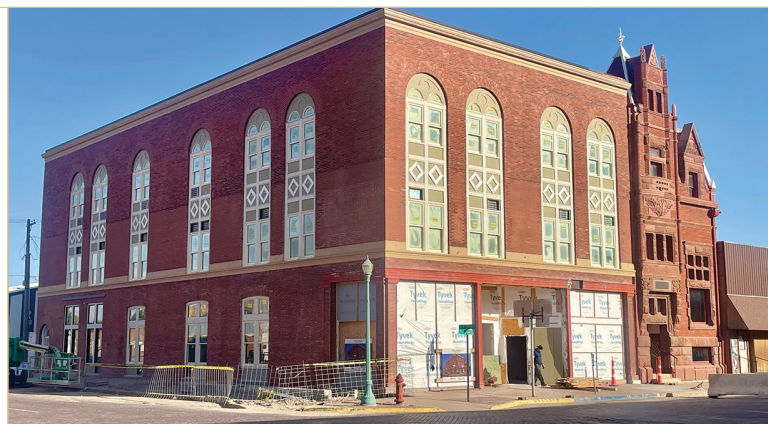
The rebuilt third floor that was lost to fire in 1961 is now overlaid with brick, and additional ornamentation has been added to the exterior facade to recreate the building's original features.
