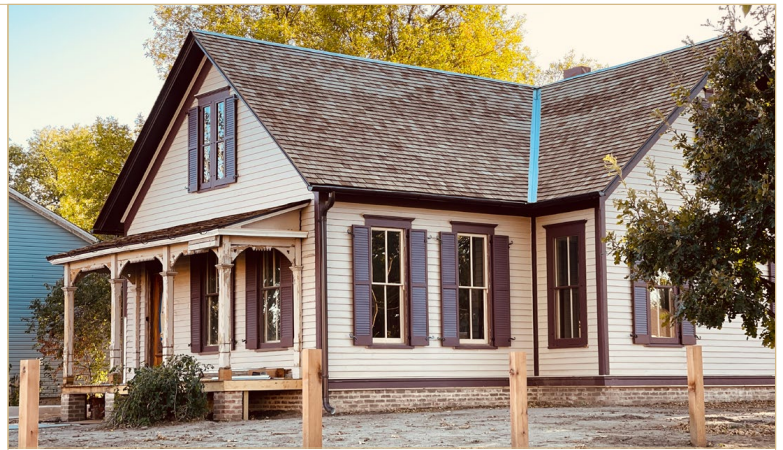
The long-awaited reopening of the Willa Cather Childhood Home will occur in December following completion of electrical upgrades, porch refurbishing, and recreation of the wood picket fence that was present during the Cather family's residency.
