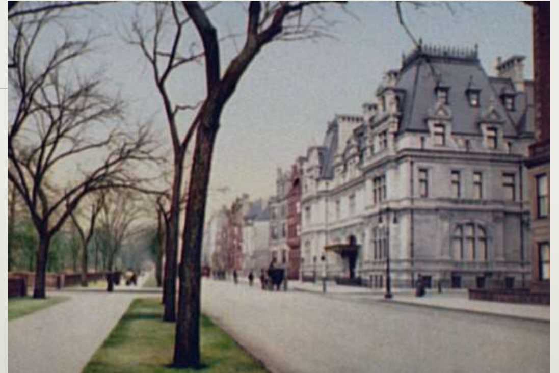
Fifth Ave. mansions, where millionaires lived
