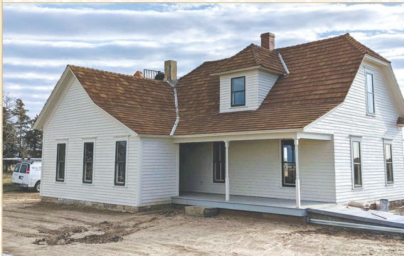
The Pavelka Farmstead following exterior restoration efforts.
