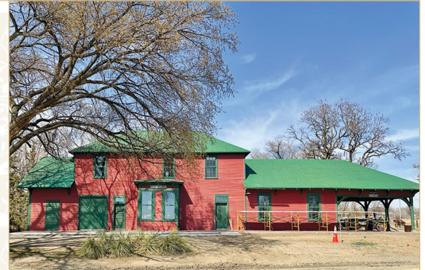
The restored facade of the Burlington Depot.
