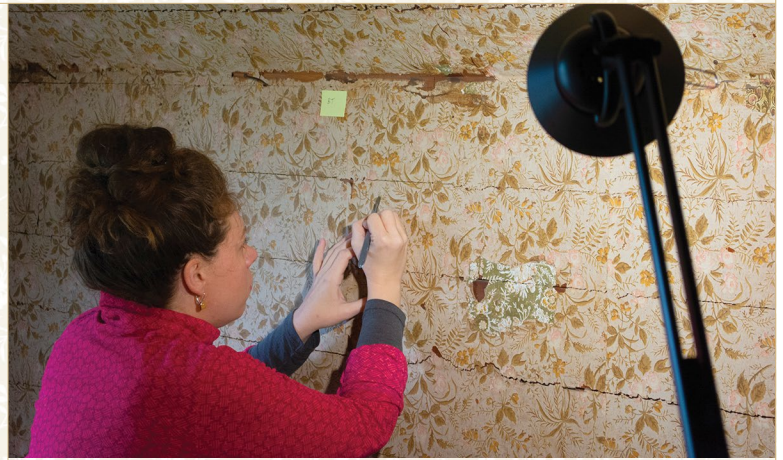
Paper conservator Hilary LeFevere carefully cleans and evaluates the original wallpaper in Cather's childhood bedroom, uncovering areas where light damage has not affected the period colorways.
