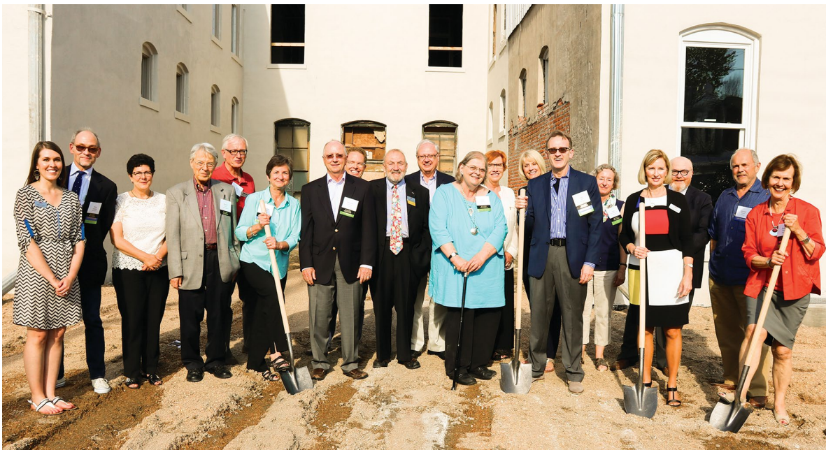
The first stage of construction already under way, the leadership of the Willa Cather Foundation and special guests got into the spirit of things with a ceremonial groundbreaking.
