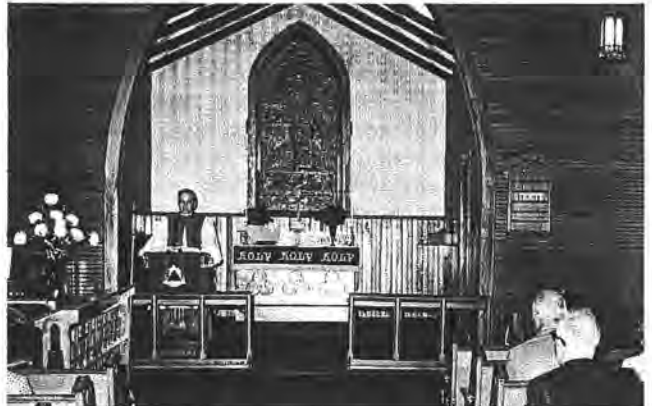
The sanctuary gleams in the soft light of the stained-glass windows which have been repaired and fitted with protective outside diffused glass.
